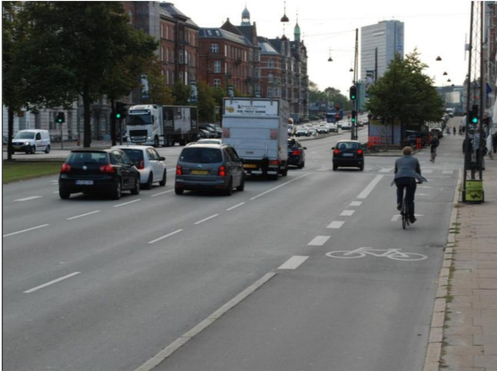
Figure 11. Example of a truncated bike lane in Denmark (Source: [Danish Road Directorate](#))
